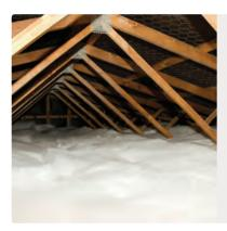
CEILING BLANKET Soft roll form blanket installed in roof cavities to cover the ceiling, including the joists. Can be double layered to achieve higher R-values.
